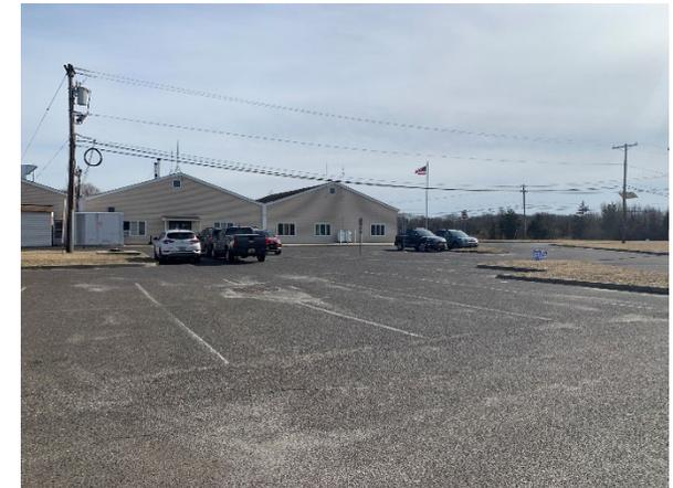
Rain gardens can be installed south of the building and pavement sections to capture, treat, and infiltrate the stormwater runoff from the buildings and roadways. The center of the parking lot can be converted to pervious pavement to promote stormwater infiltration. A preliminary soil assessment suggests that more soil testing would be required before determining the soil's suitability for green infrastructure.
